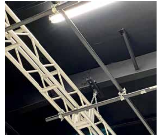
GRID ROOF ATTACHMENT
